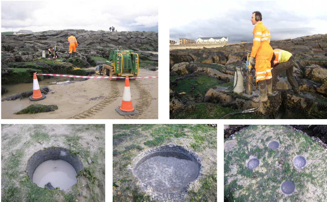
Figure 4: Habitat enhancement: drill-cored rock pools at Tywyn. (Firth et al. in press, Coastal Engineering, Photos L. Firth)
