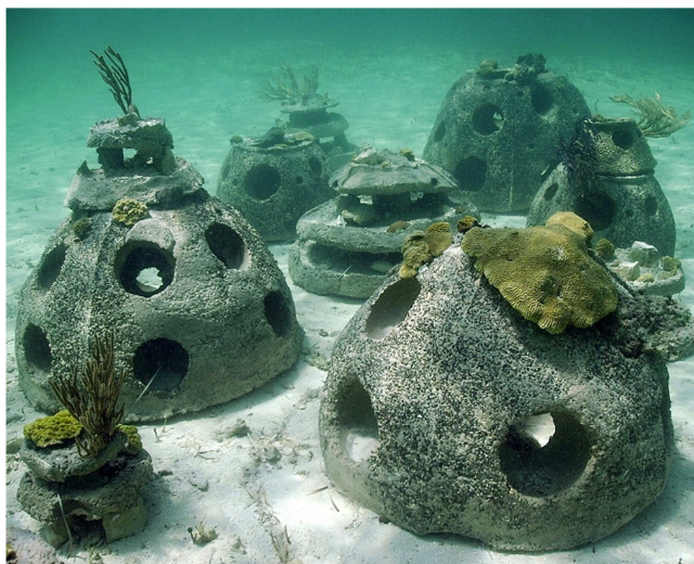
Figure 6. Pre-fabricated reef blocks; a) Reefballs are used to promote biodiversity ( www.reefball.org ); b) BIOBLOCK (Firth et al. 2012)
