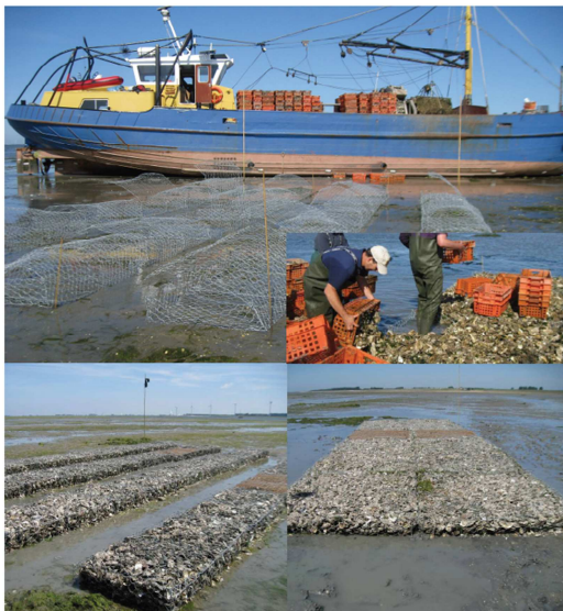
Figure 7: Shell filled gabions in intertidal areas to prevent erosion.
