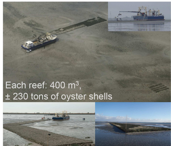
Figure 7: Shell filled gabions in intertidal areas to prevent erosion.
